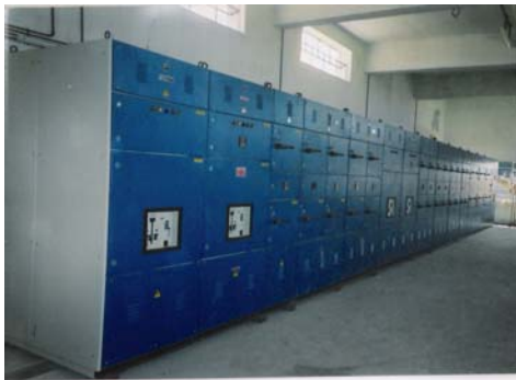
Intelligent Motor Control Centre (IMCC)
