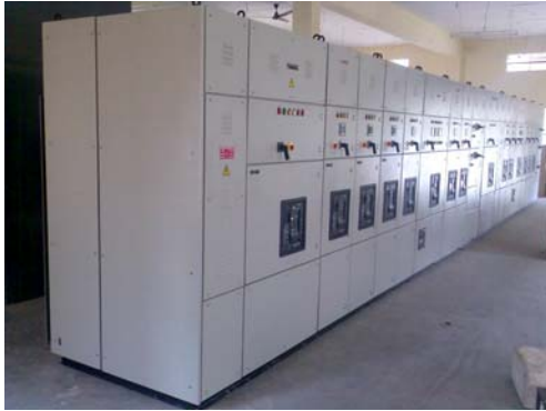
Double Busbar Changeover Panel
