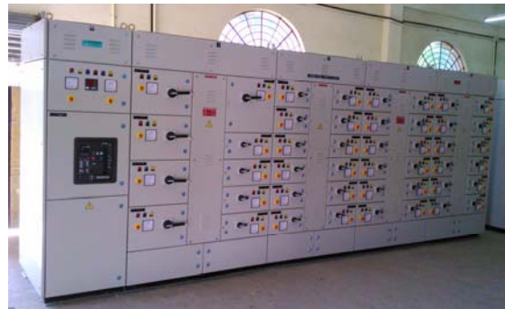
Intelligent Motor Control Centre (IMCC)
